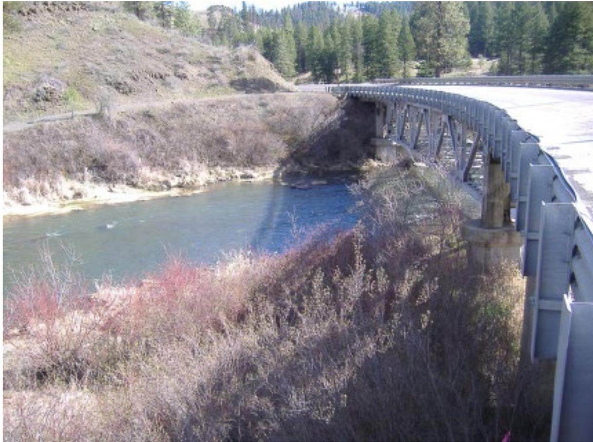
Existing Bridge was a 285-foot (ft) long bridge. The approach spans consist of reinforced concrete deck girders and the center span is a 150-ft long truss and includes 1 bent within OHW and 1 partially within the OHW
