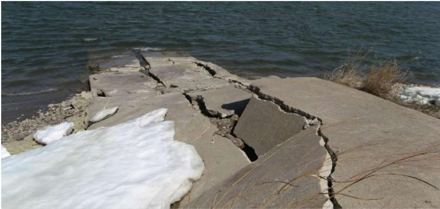
**The Sunshine Bottoms boat launch on the Lewis & Clark Reservoir in Nebraska suffered from freezing and thawing breakages before it was reconstructed with a concrete ramp mat.**
