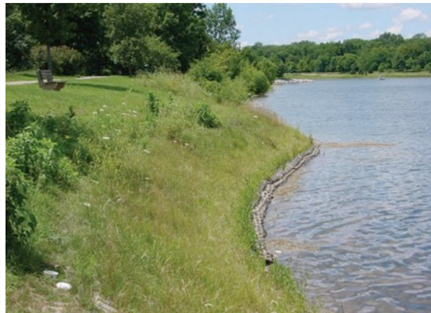
Same site with fully vegetated concrete block/geotextile installation completed
