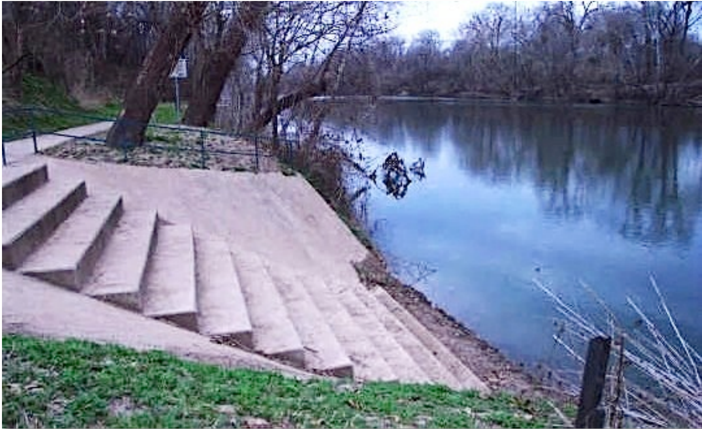
Steep shoreline grade prevents site from being entirely accessible: concrete stairs provide access to base of an accessible trail.
