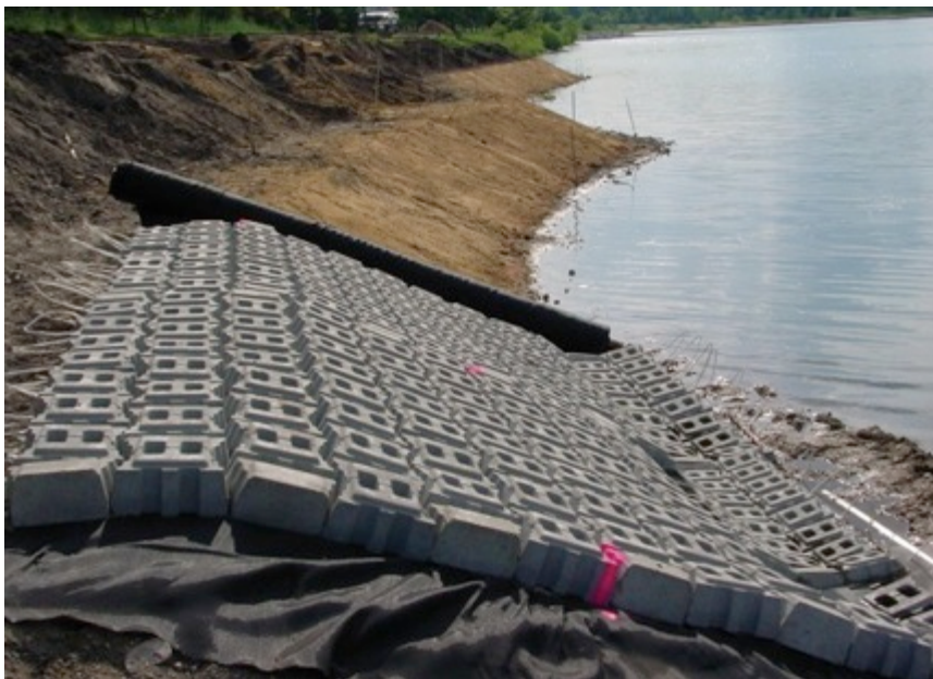
Articulating concrete block installation with geotextile fabric
