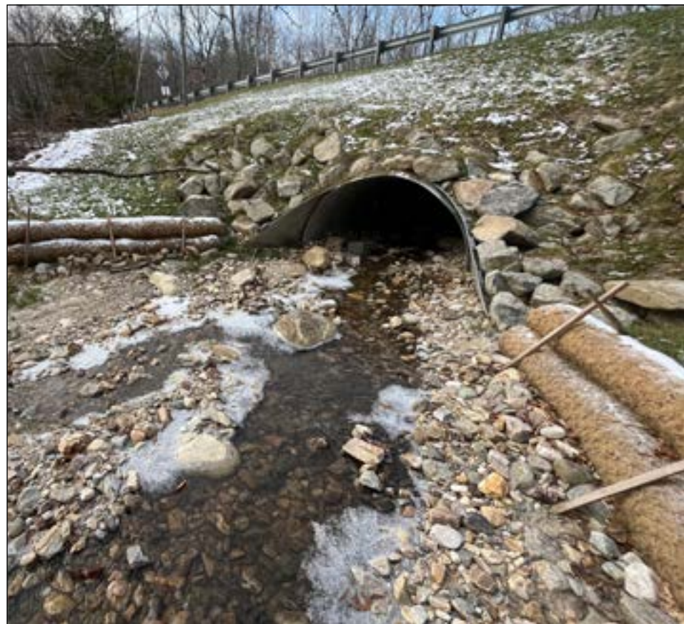
Completed Culvert Replacement on the Westfield River: A culvert designed to improve flood resilience and restore aquatic connectivity for fish and wildlife. Photos: Andrew Petit de Mange
