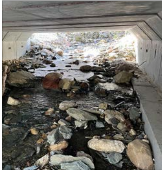
Completed Culvert Replacement on the Westfield River: A culvert designed to improve flood resilience and restore aquatic connectivity for fish and wildlife. Photos: Andrew Petit de Mange
