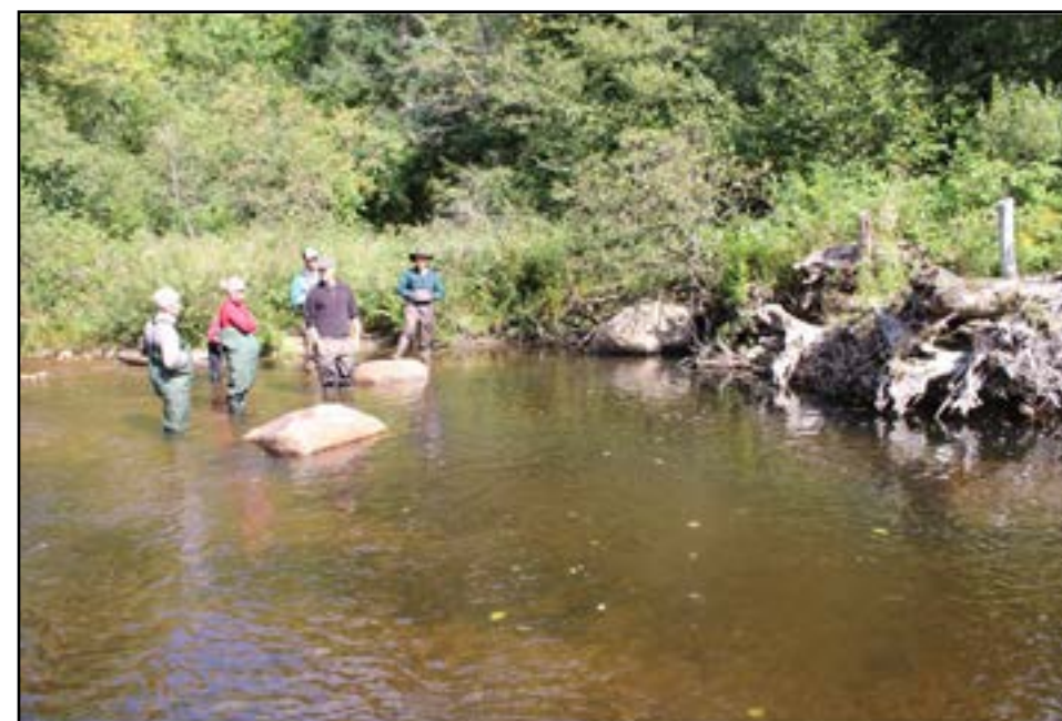
Figure 2. Participants on the northern New Hampshire field trip observe an engineered log jam on Nash Stream built to encourage pool formation and the redevelopment of meanders on an artificially straightened channel heavily impacted by log drives decades ago.
