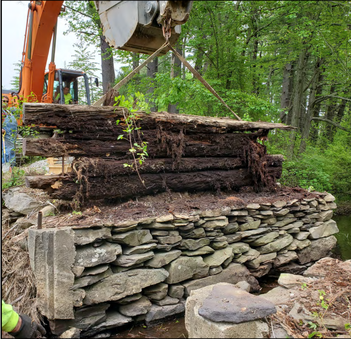
Removing rotted base of bridge
