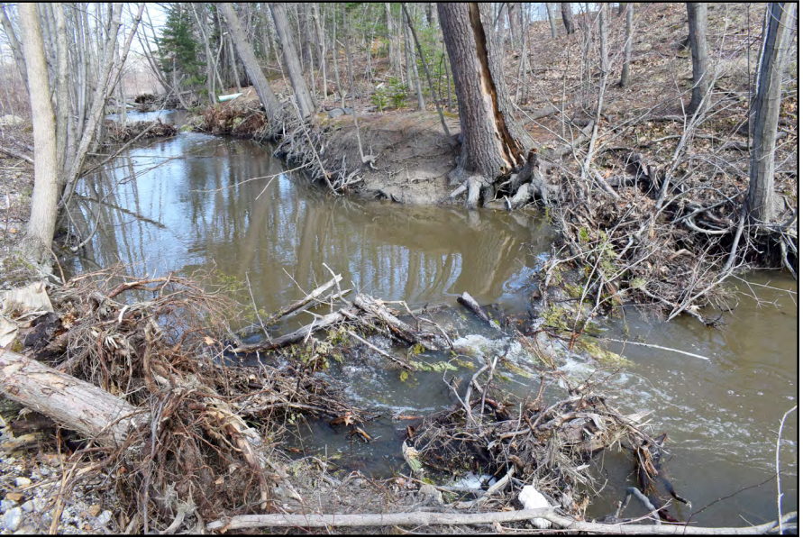
Figure 3. Constructed full-spanning log jam in restored reach of Long Creek showing flow complexity created as flow passes over and through the structure five months after construction. Two other constructed log jams are visible in background.
