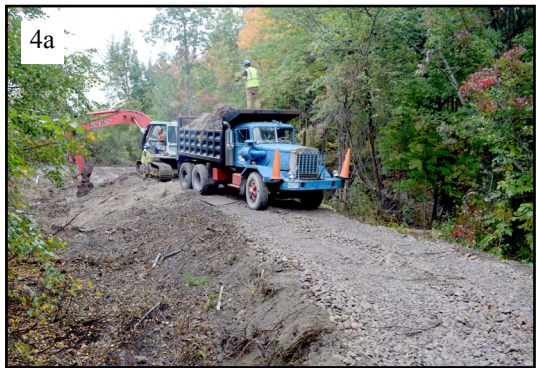
Figure 4. Long Creek restoration included a) removal of a stormwater retention berm to b) reconnect a portion of the floodplain.
