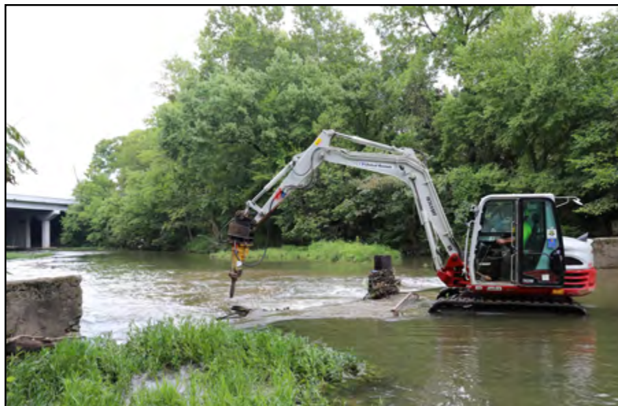
Excavators were used to break apart and remove obsolete dams in Mill Creek.
