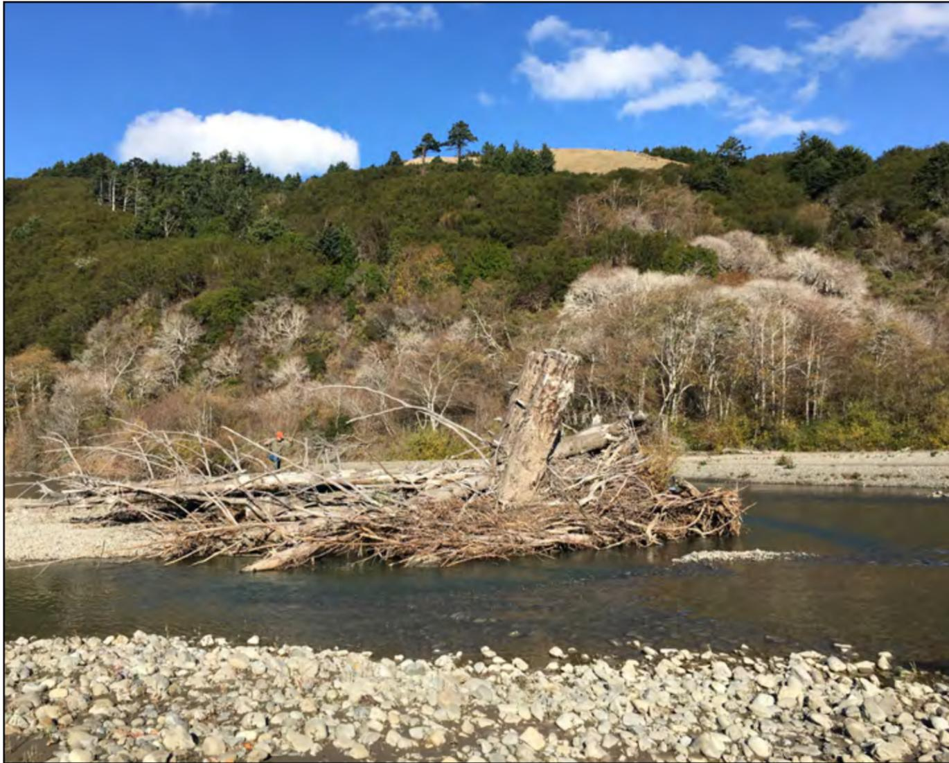
The structure known as “Woodzilla II,” composed of trees delivered by helicopter and naturally accumulated debris, protects an existing mid-channel island. A deep pool on the upstream side of the structure provides complex habitat for salmon and steelhead. (Photo: Zane Ruddy, BLM)
