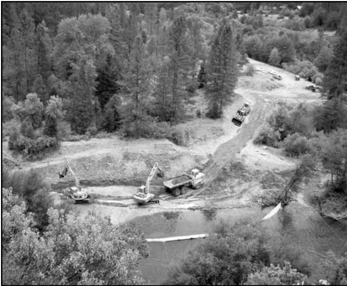
Restoration sites vary in their objectives, approaches and size. A 2009 restoration site at Sawmill on the Trinity River involved lowering topography to create a flood plain to increase fishery habitat during prescribed flows.
