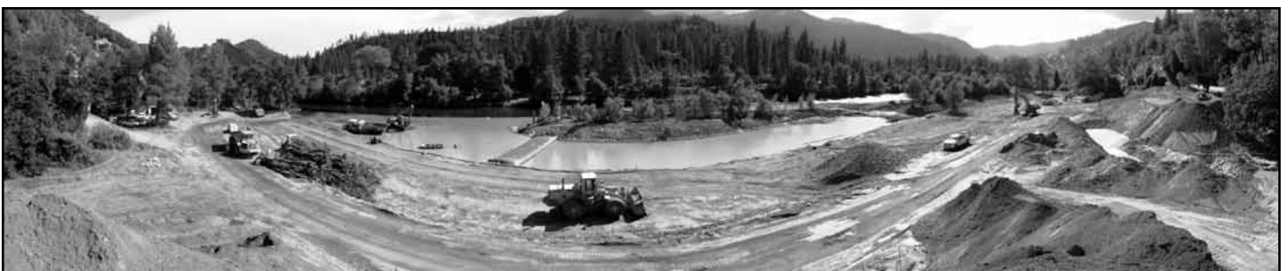
Above: Pre-construction riverside habitat along the single channel of Trinity River at Wheel Gulch. Below: The Wheel Gulch site during construction of a split flow channel around an island that includes part of the original bank, a low flow side channel, an alcove, and a habitat enhancement channel to reconnect the existing Wheel Gulch drainage to the mainstem.
