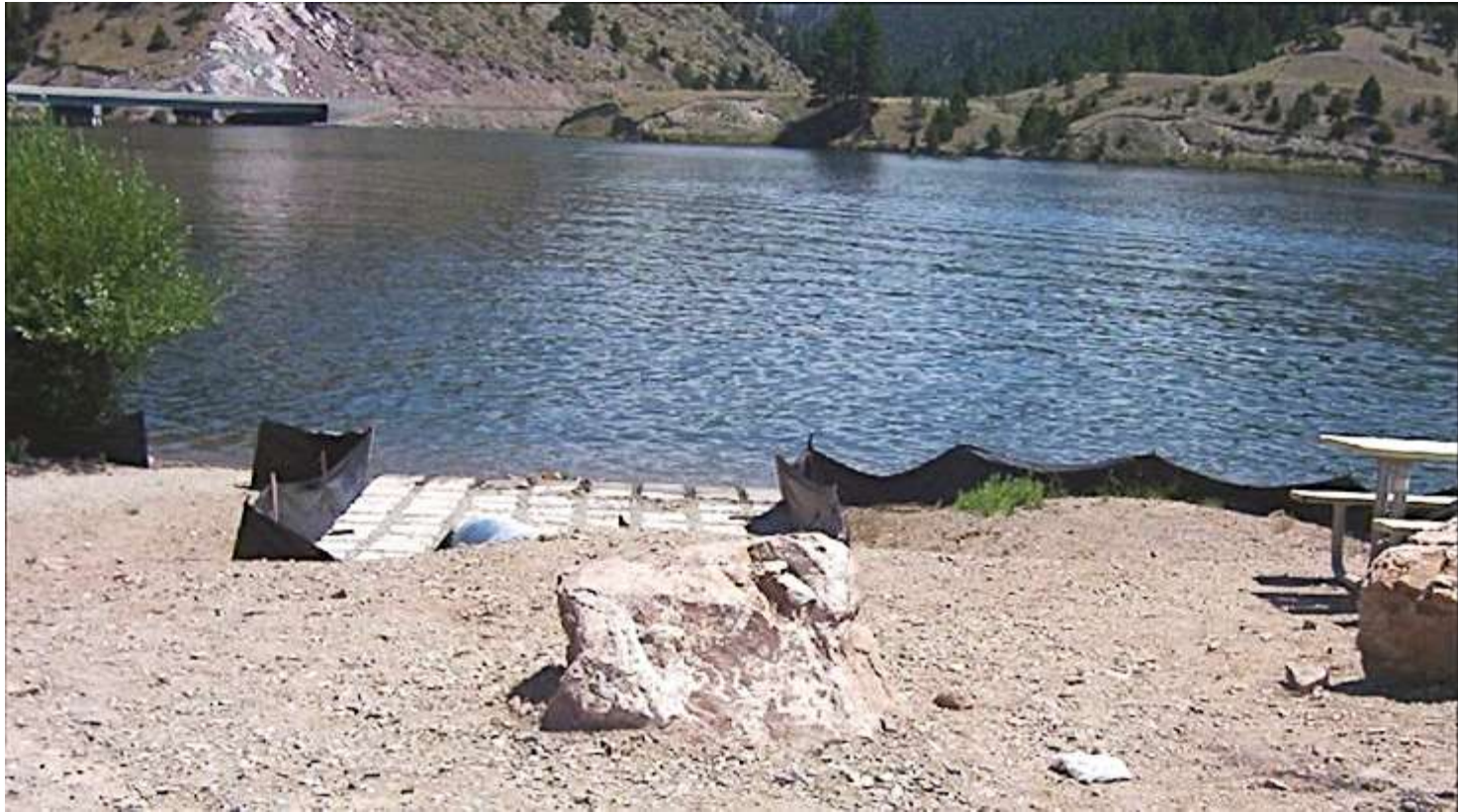
An articulated concrete launch helps to protect against the effects of erosion while providing paddlers with a separate access site from heavy boat traffic.
