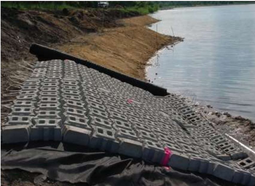
Articulating concrete block installation with geotextile fabric
