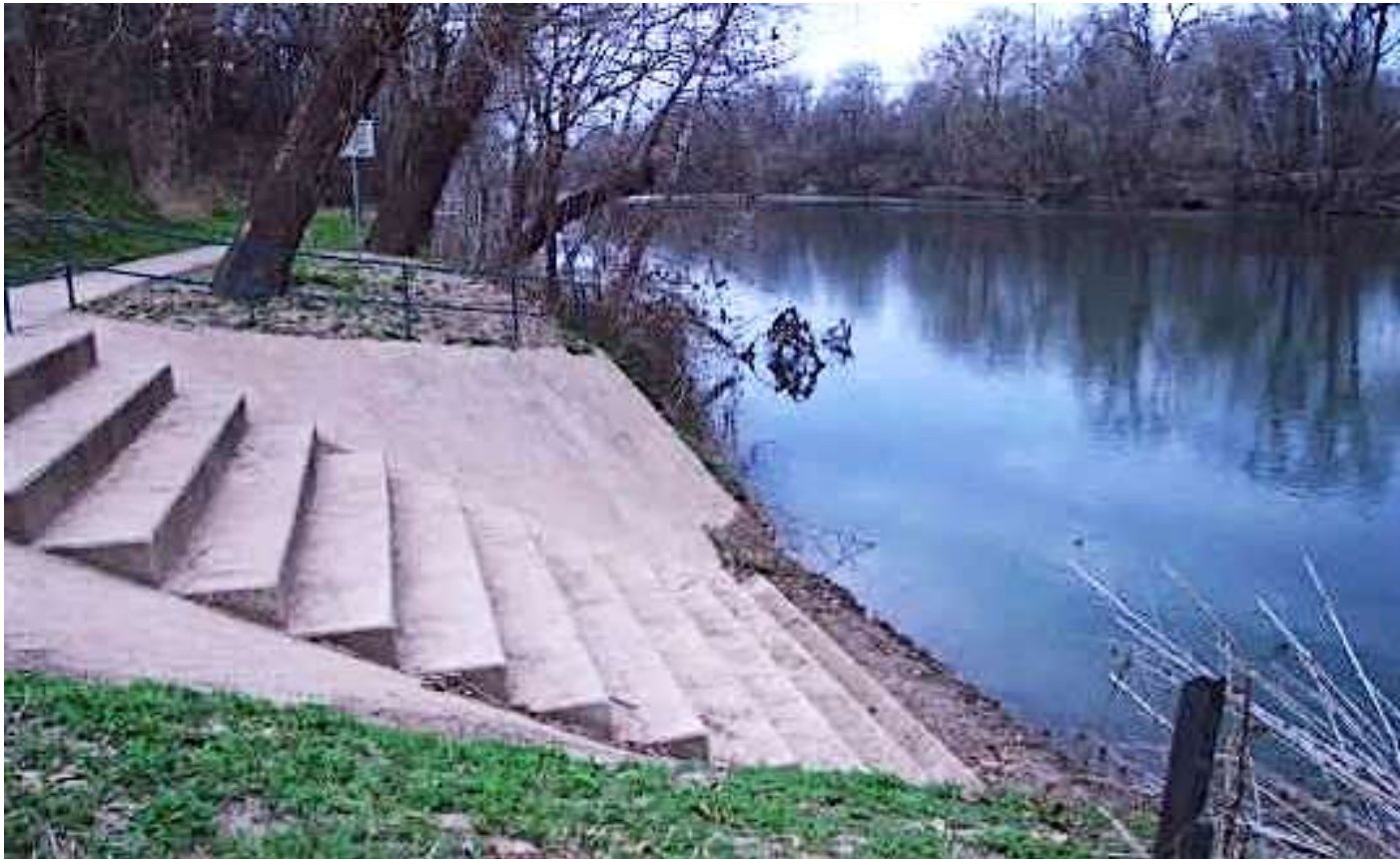
Steep shoreline grade prevents site from being entirely accessible: concrete stairs provide access to base of an accessible trail.
