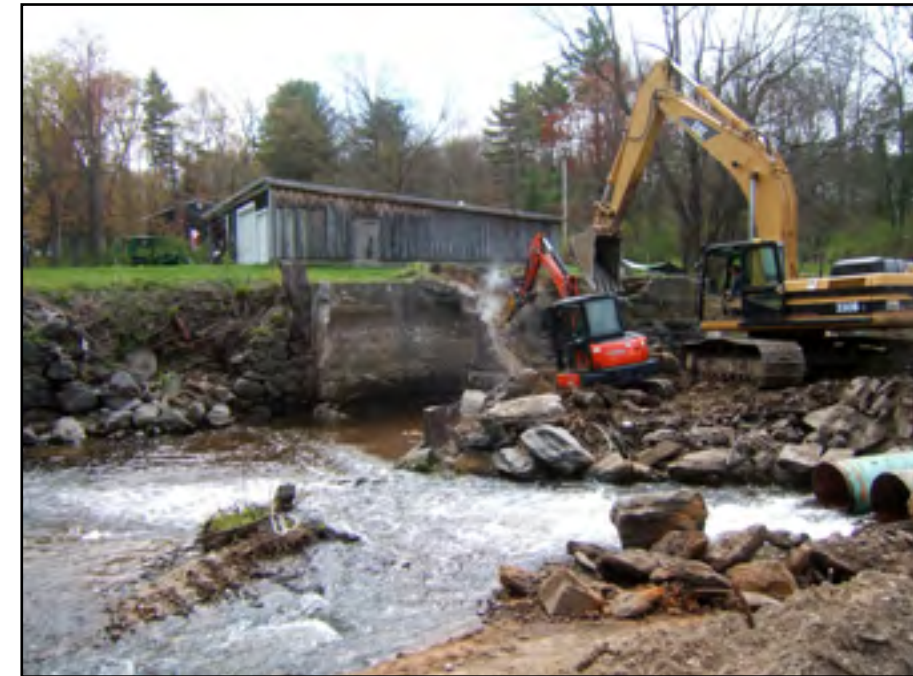
Above: Removing spillway.
