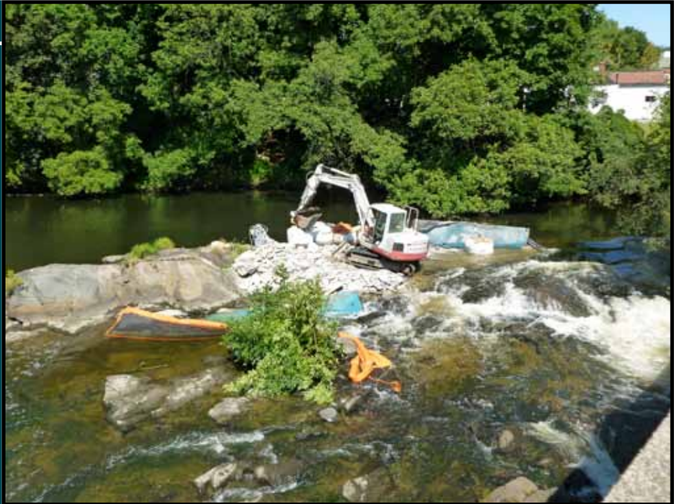
Excavator at work removing Pawtuxet Falls Dam.
