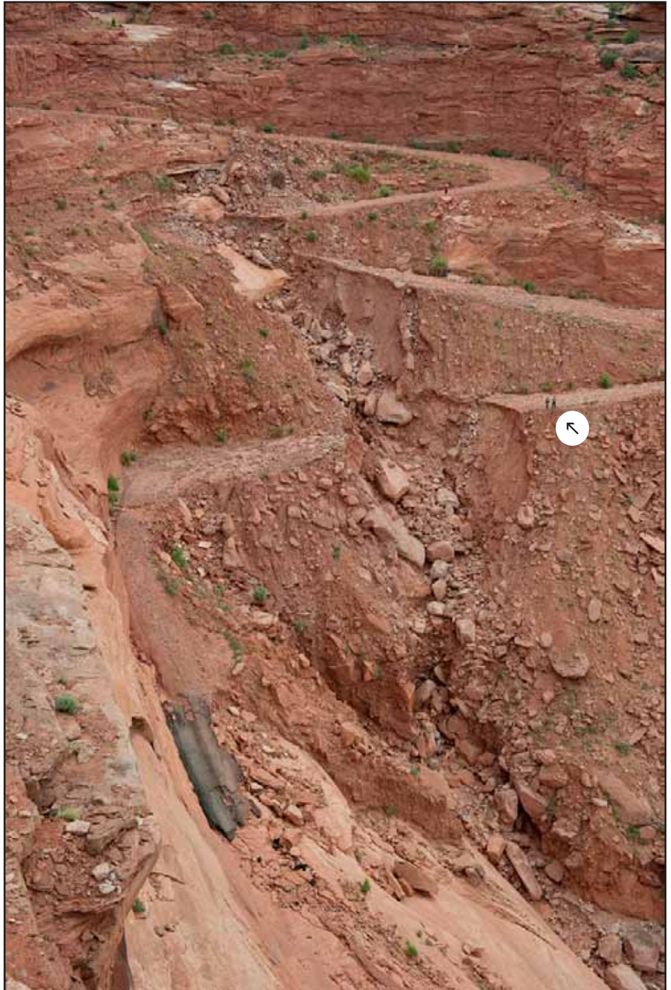
On August 19, 2010, severe thunder storms caused a major rock and mud slide and washed out the road to Mineral Bottom, the traditional boat take-out for the Labyrinth Canyon segment of the Green River. (Note arrow and people on road.)
