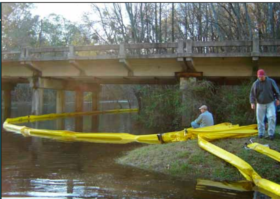
Containment booms being installed by state contractor and DHEC staff. Photo: SC DHEC
